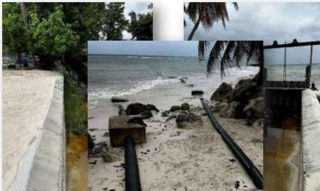
Figure 108: Sluice gate and channel at FV-07. The structure appeared inoperable during the August 2026 field visits, with low/stagnant water and restricted apparent wetland–coastal exchange.
