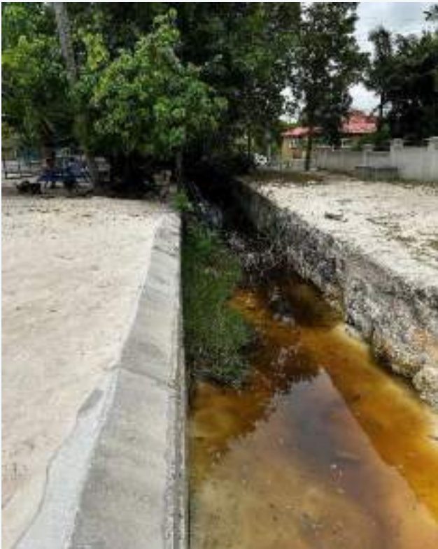
Photo 57 Water Channel leading to the Sluice Gate
