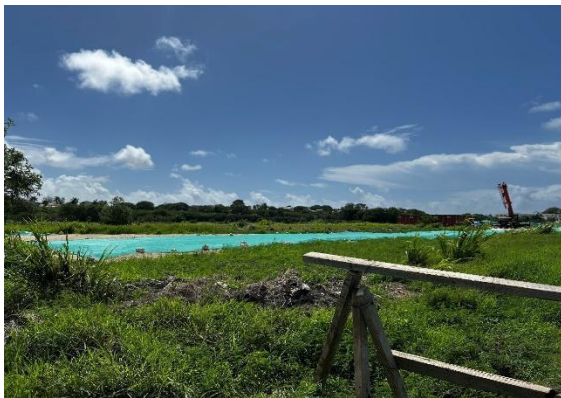
Figure 2: Project Interface - Site for the new Water Reclamation Facility
