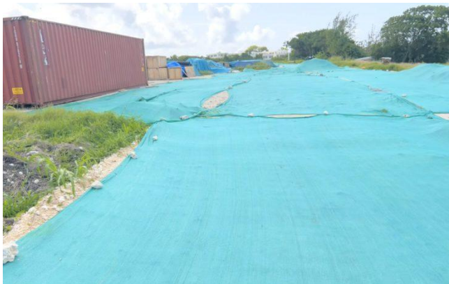
Figure 4: Project Interface: Shade cloth being used for dust mitigation
