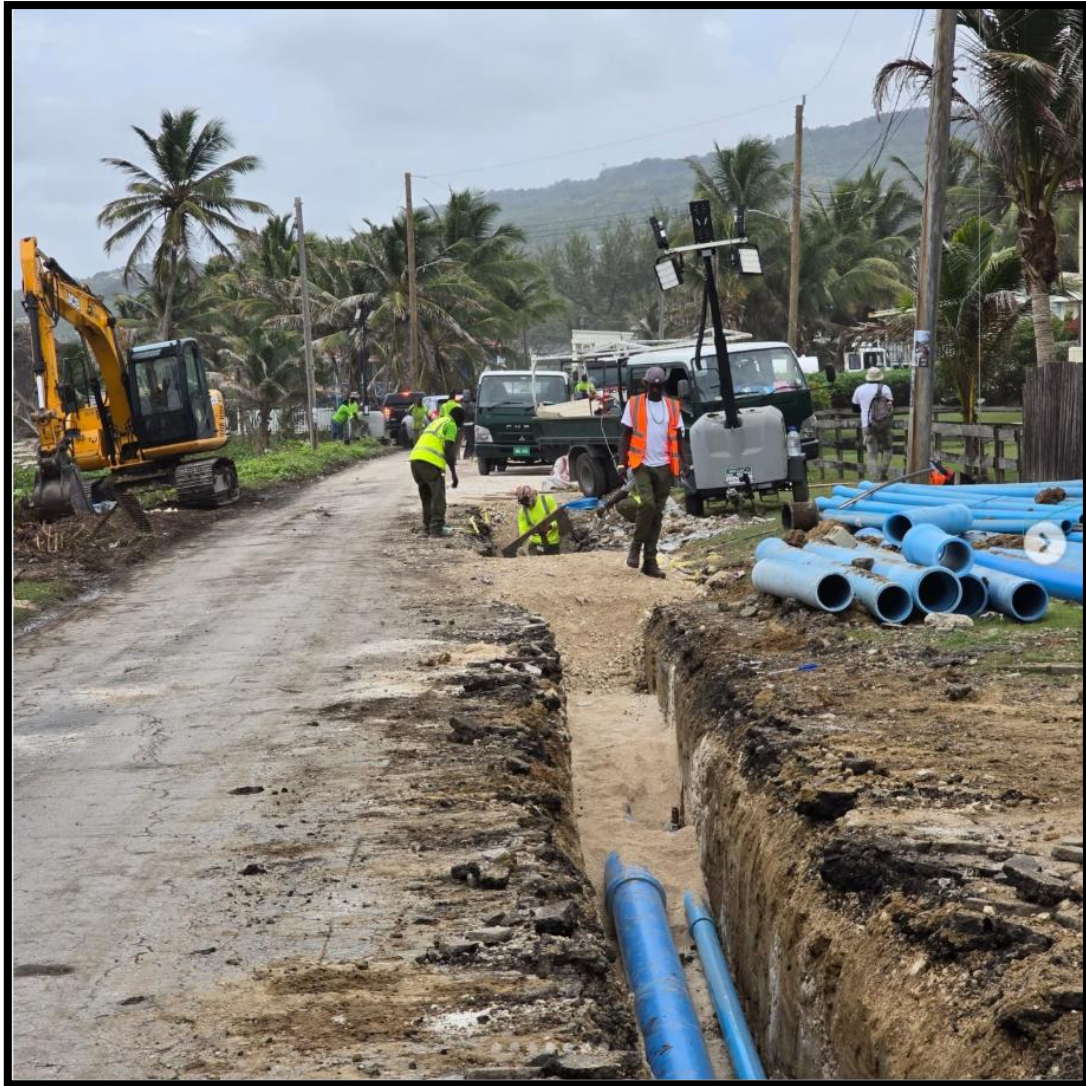
Figure 3. Similar mains replacement work by BWA on Ermie Bourne Highway. Source: https://www.instagram.com/p/DJOpVbHxocQ/
