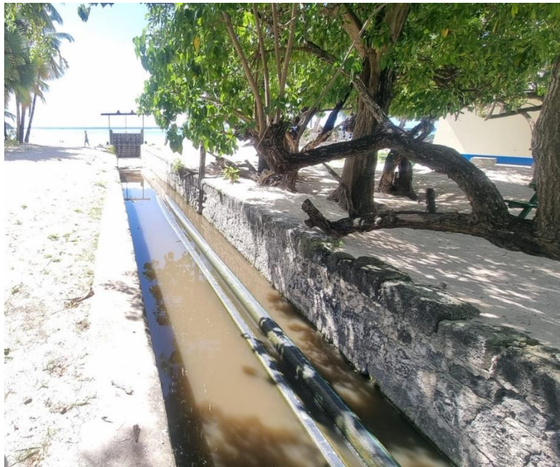
Figure 5-34: Graeme Hall Swamp Sluice Gate
