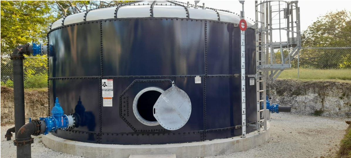
Figure 4- Storage Tank at Ellerton, St. George
