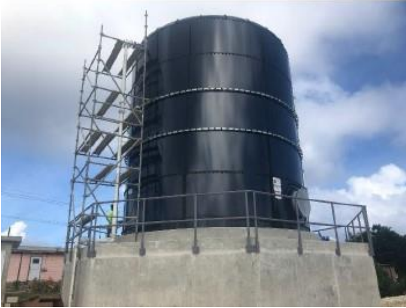
Figure 1- Storage Tank at Mount Stepney, St. Peter
