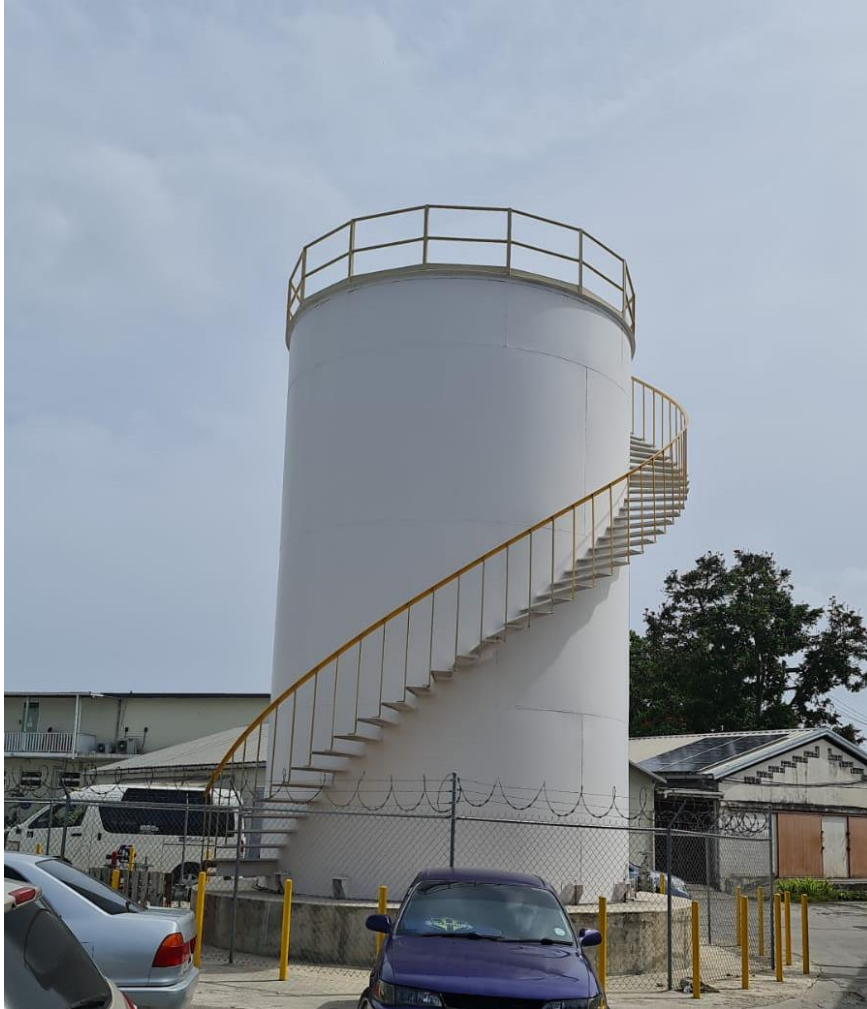
Figure 6- existing 50,000 gallon tank to be replicated at Queen Elizabeth Hospital
