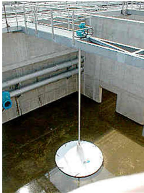
Figure 8-10: Bioreactor – Anoxic Zone
