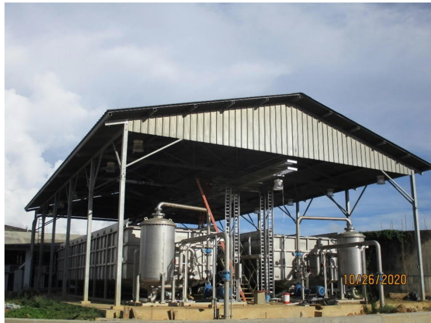
Figure 8-13: Dissolved Air Flotation (DAF) – Sludge Thickening (Ref: SFWWP, Trinidad)
