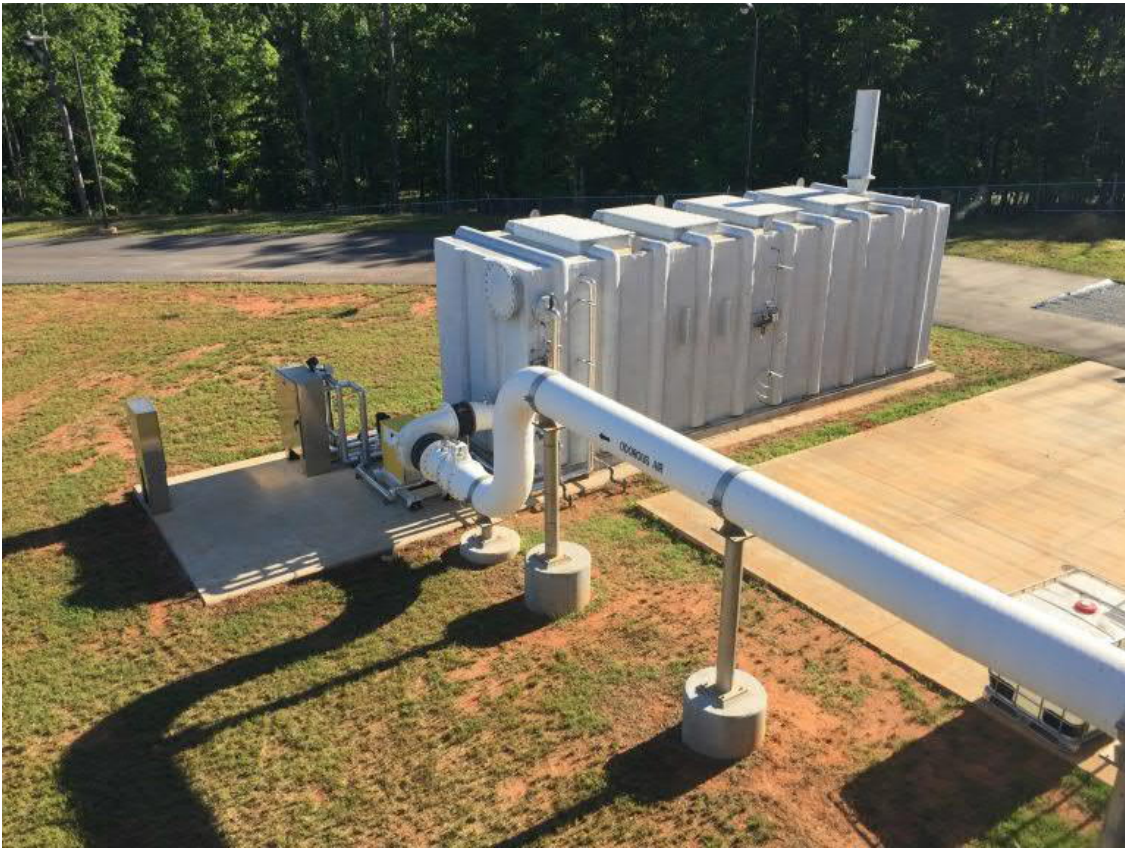
Figure 8-5: Pre-Engineered Odour Control Unit (Source: Biorem)
