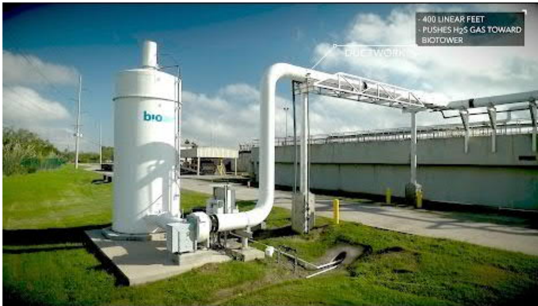
Figure 8-7: Pre-Engineered Odour Control Unit (Source: BioAir)
