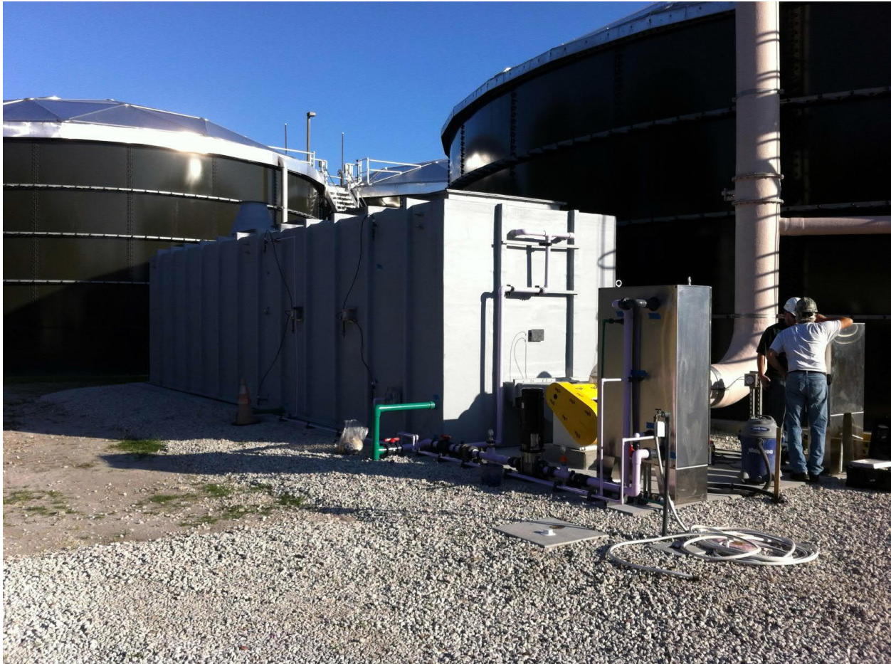
Figure 8-4: Pre-Engineered Odour Control Unit (Source: Biorem)
