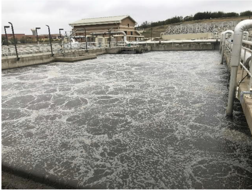
Figure 8-9: Bioreactor – Aeration Zone (Diffused Air)
