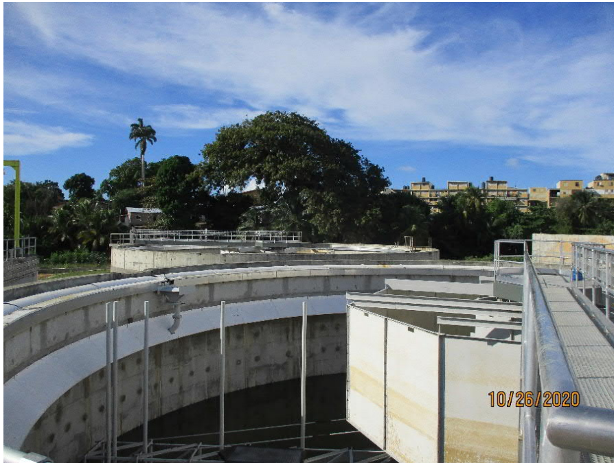
Figure 8-11: Secondary Clarifiers (Ref: SFWWTP, Trinidad)
