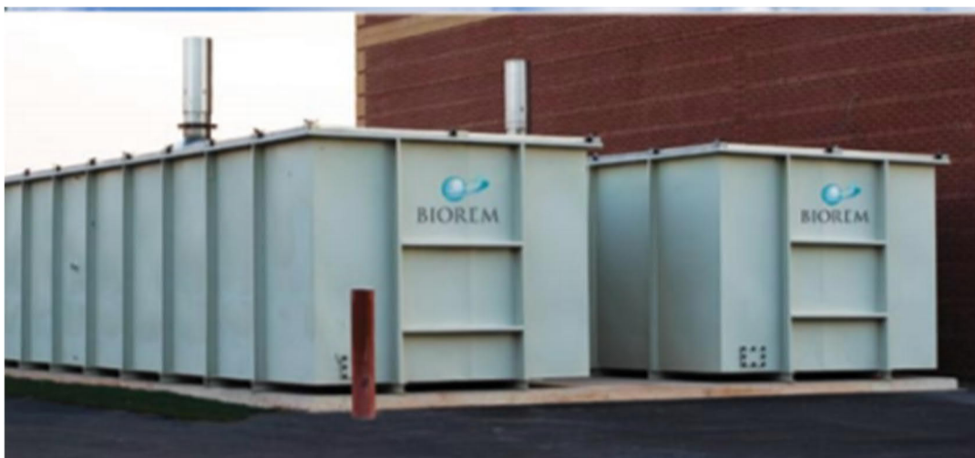
Figure 8-6: Pre-Engineered Odour Control Unit (Source: Biorem)
