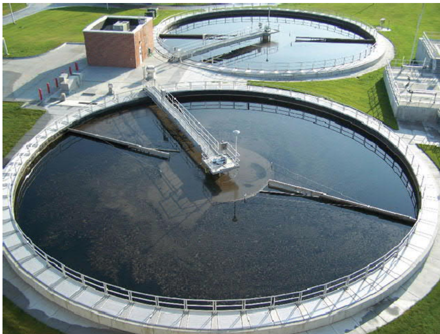
Figure 8-12: Secondary Clarifiers (Ref: USA)
