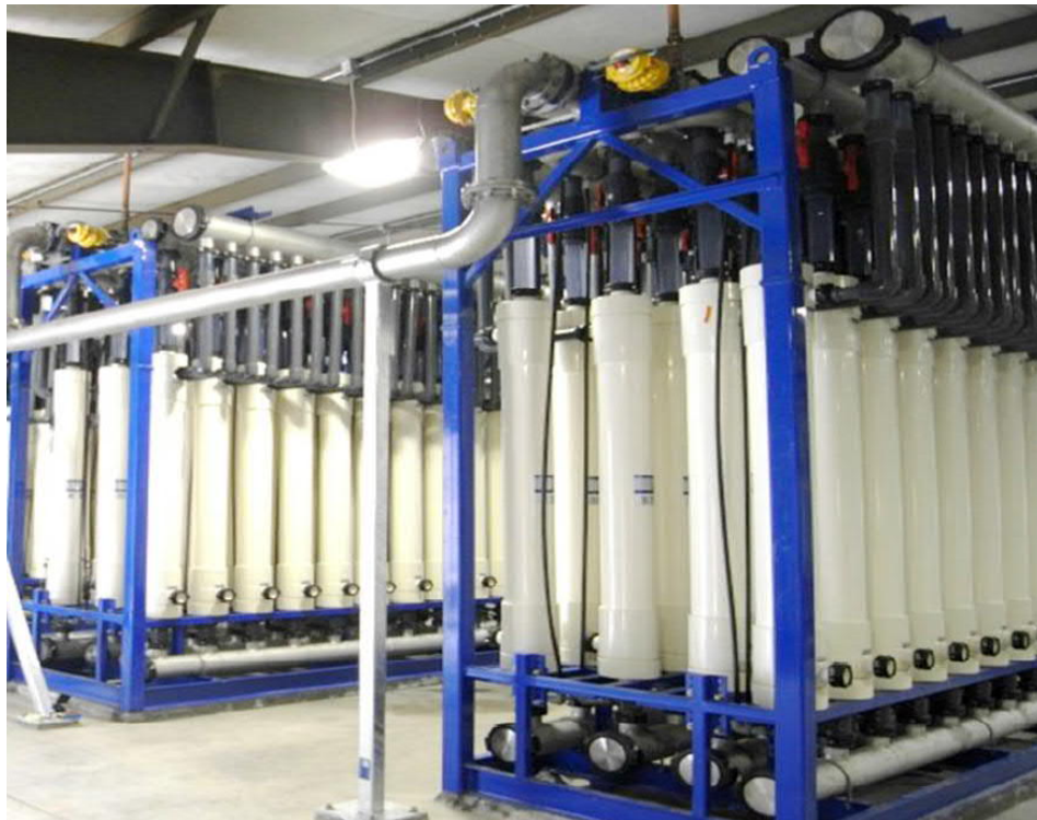
Figure 8-24: Example of MF/UF Skid (H2O Innovation)
